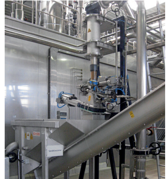
LOHSE hydrocyclone plant 200K.
