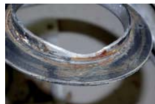
Wear of the flange ring
